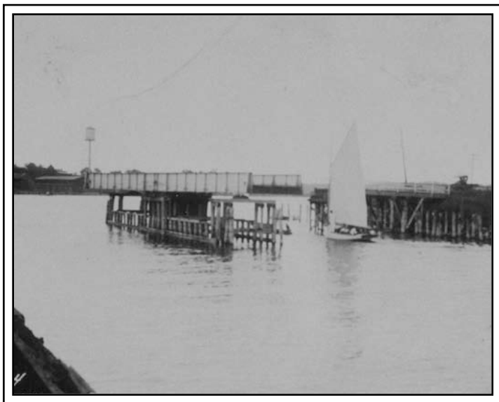
A view of the swing bridge opened to allow the passage of the sailboat. That's the water tower in the background.
