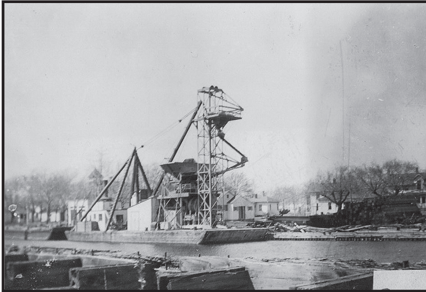
Reconstruction of the channel including dredging by this machine took place in 1938.
