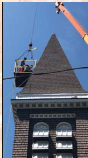
A crane and a work platform was used to reshingle the steeple.
