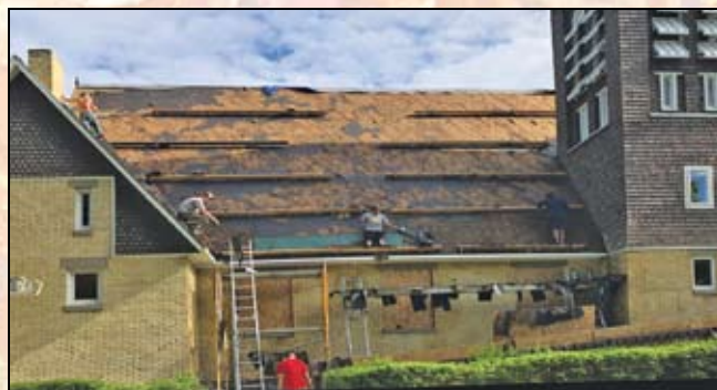
Preparation is a major part of roofing. Peffer's crew laboriously ripped off old shingles and tar paper right down to the roof boards.
