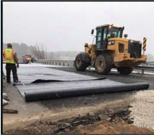
The Longbridge Road becomes passable much to the delight of residents along Wayne Road and along the lake. Here, the crew is laying down heavy sheeting material to stabilize the soil.
