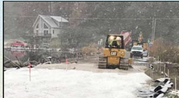
Heavy equipment spread lots of gravel to raise the roadbed a couple of feet.
