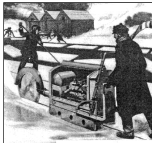
Icing became more efficient with the use of powered ice saws.
