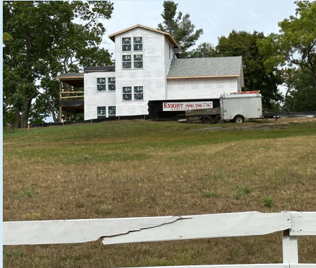
Houses going up on the old Nickerson Inn property
