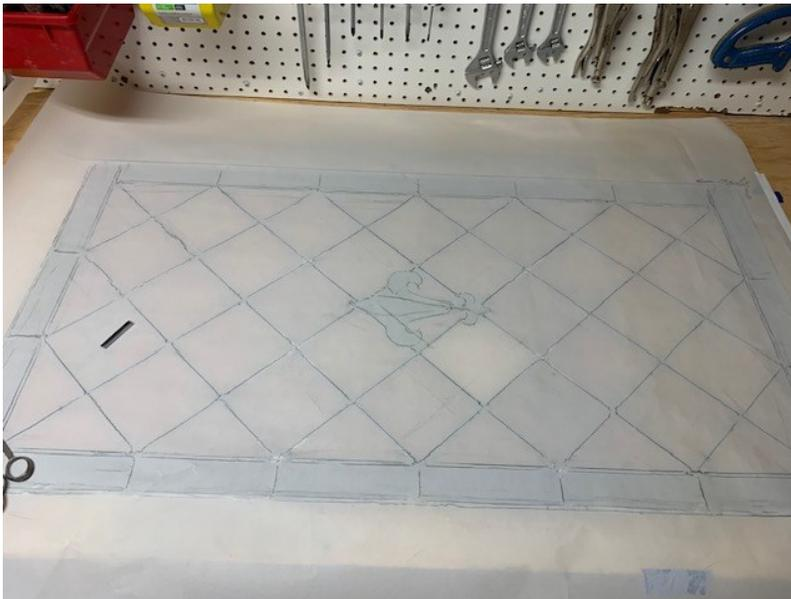
Tom began the process of restoring the window panels by delicately removing the windows. Each of the three windows had to be removed completely, transferred to Tom's home, traced to capture the pattern and disassembled piece by piece. Each window has 74 pieces.
