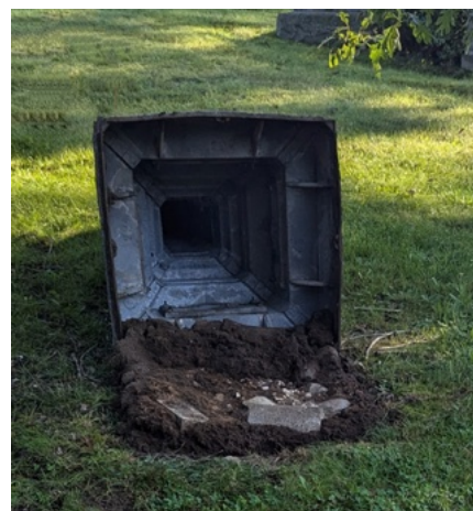
Interior view of a white bronze monument, taken during a Cemetery Preservation workshop at Mountain Home Cemetery in Kalamazoo, summer 2024
